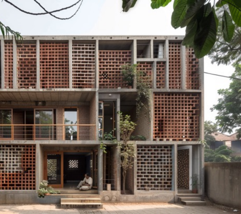
Structures using Fly ash bricks
